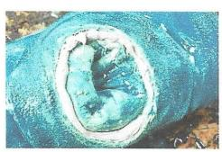
Silicate resin was evenly distributed over the exterior of the full-wrap for additional adhesion to the host pipe.
