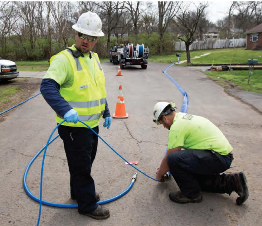
BLD Services Superintendent P.J. Boihem (left) and Brent Faust work together to prepare a lateral liner for installation.
