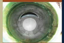
Providing a structurally sound service lateral with a watertight seal at the connection
